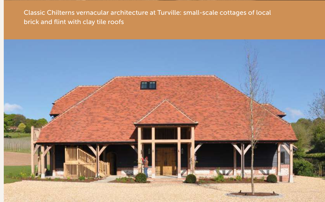
The Chilterns Conservation Board runs the Chilterns Building Design Awards with the Chiltern Society to encourage and recognise good design. This new build Winery at Hundred Hills Vineyard, South Oxfordshire won the latest awards
