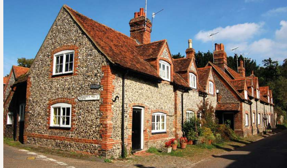
Classic Chilterns vernacular architecture at Turville: small-scale cottages of local brick and flint with clay tile roofs
