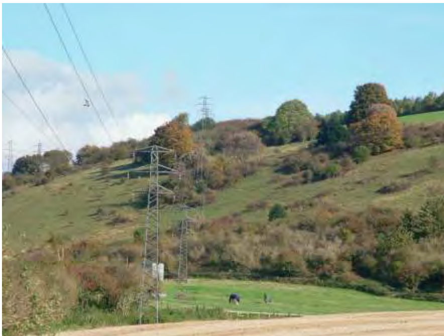
Dunstable Downs - overhead wires that are a good candidate for removal
