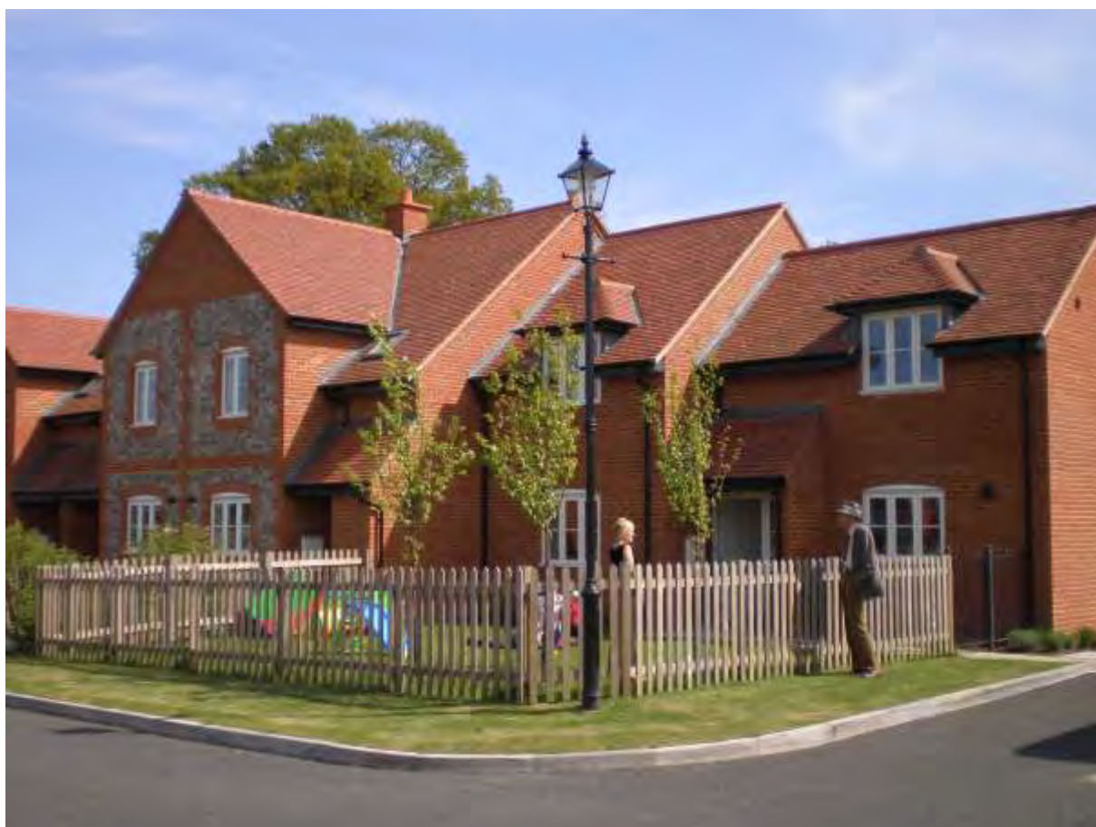
Affordable housing at Winchmore Hill, acceptable design though difficult to assess in terms of the sustainability of construction
