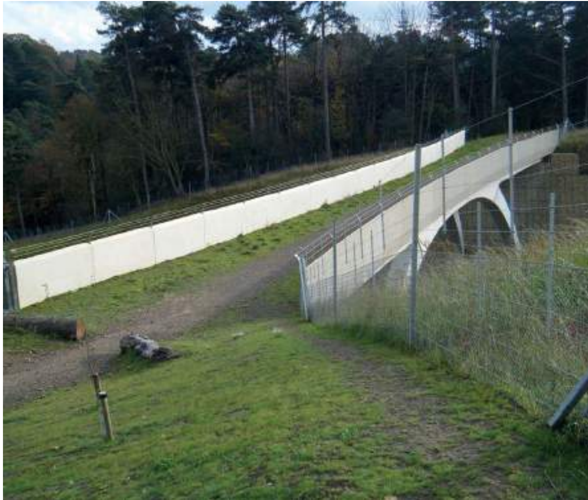
Greened pedestrian bridge, A3 Hindhead
