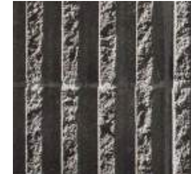
Ribbed concrete. Light and shade produces darker appearance
