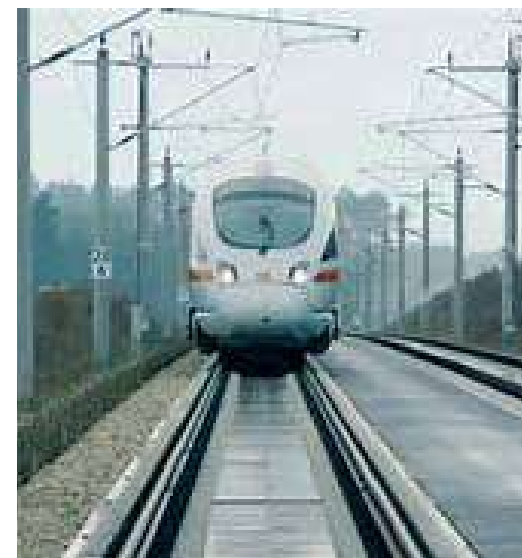
Cantilever OLE masts
