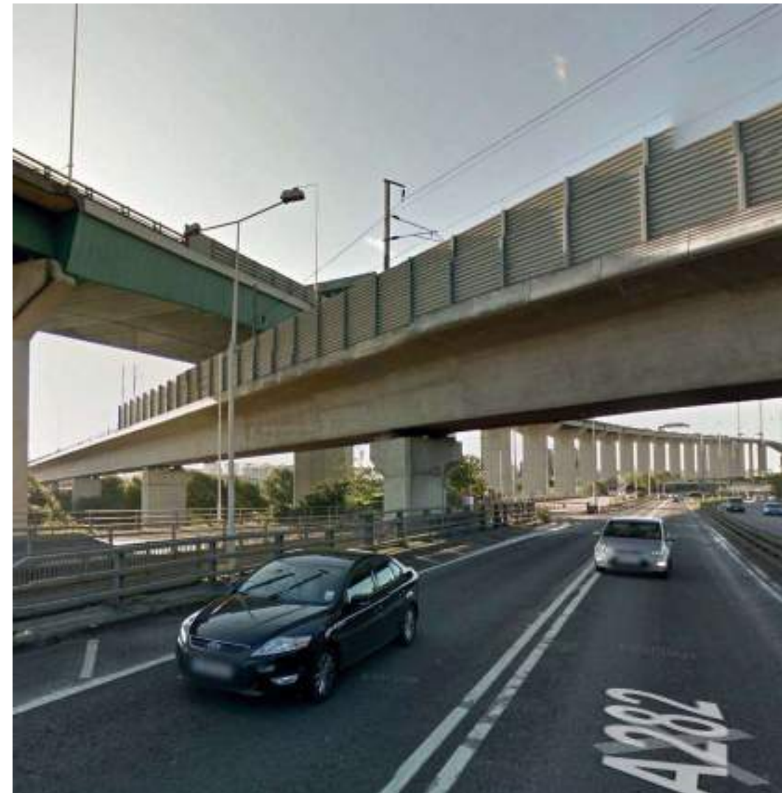
Noise mitigation at the cost of visual intrusion, HS1 crossing the M25, Thurrock
