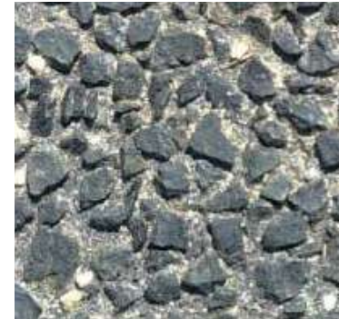
Abutments: Exposed dark coloured exposed aggregate concrete
