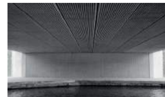
Ribbed bridge soffit, Kings Cross
