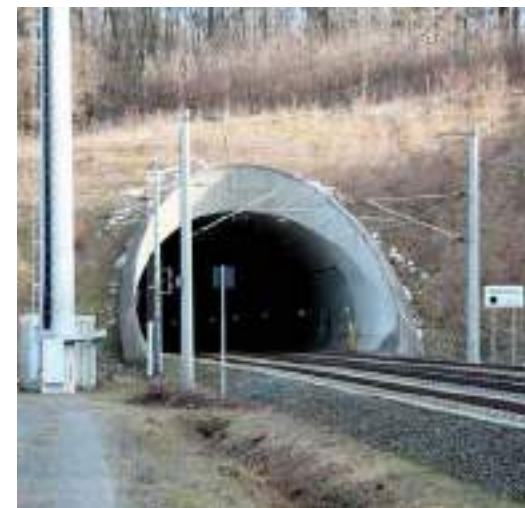
Hellenberg Tunnel, north portal (Germany)
