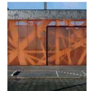
Corten artwork (potential use for Wendover South Portal noise barriers and Chiltern North portal)
