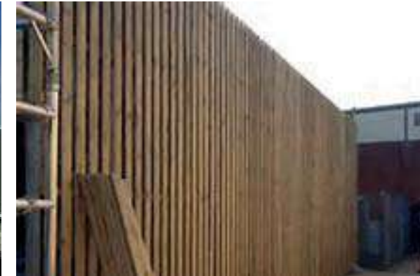
Ribbed timber barrier
