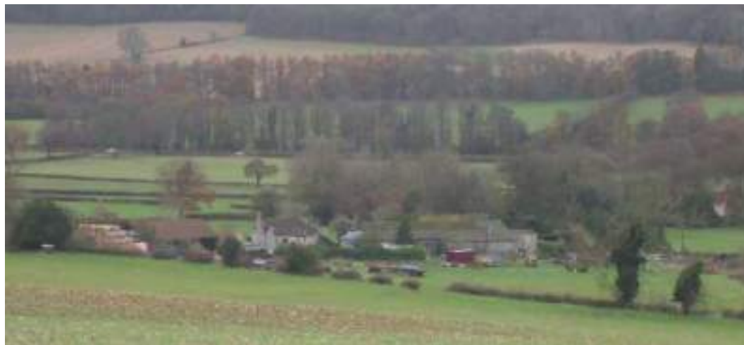
Durham Farm and the immediate context of the proposed Wendover Dean Viaduct. The farm will be demolished.
