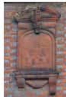
Date panel with moulded and carved brickwork (Amersham)
