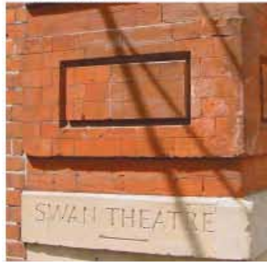
Quoins in expressed panels with rubbed and cut bricks (High Wycombe)
