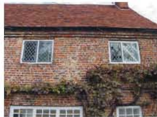
Brickwork formerly coated with limewash (Bisham)
