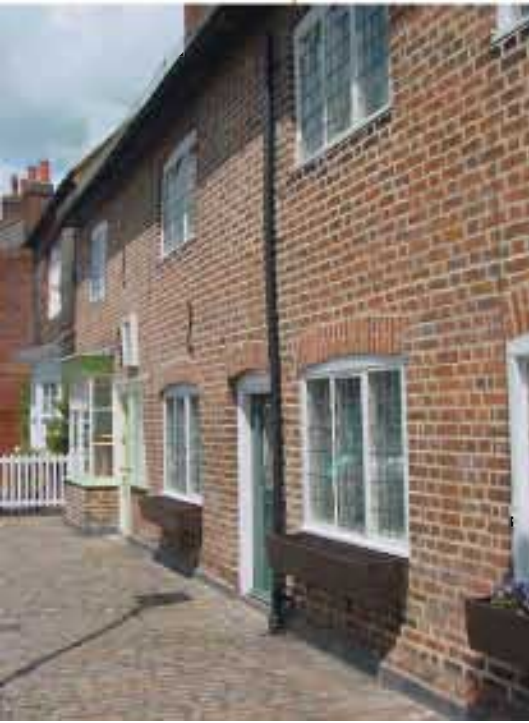
Carefully restored brickwork will enhance the street scene (Amersham)
