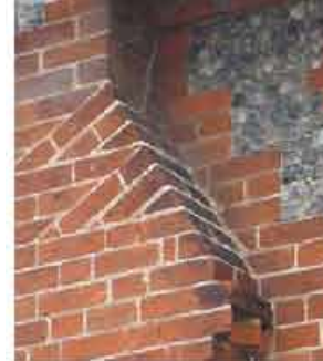
Tumbled-in brickwork
