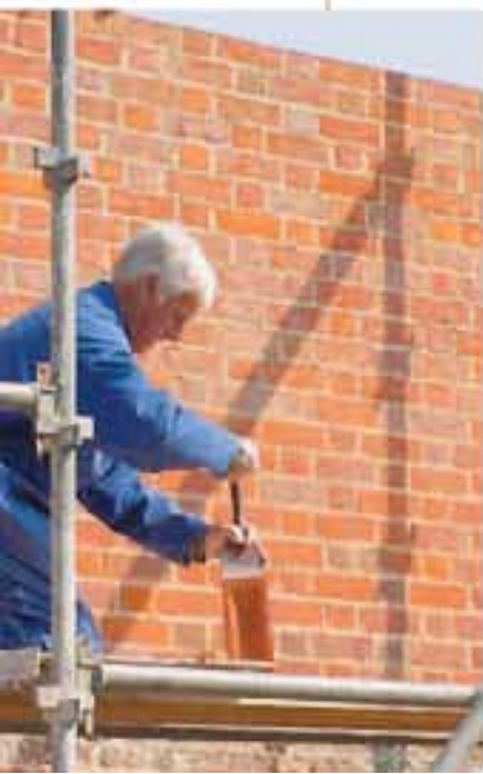
Brick wall under construction (Bradenham)
