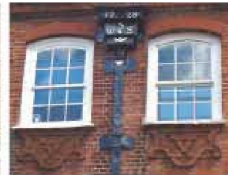
Elaborate aprons in rubbed brickwork and gauged segmental arches (Hemel Hempstead)
