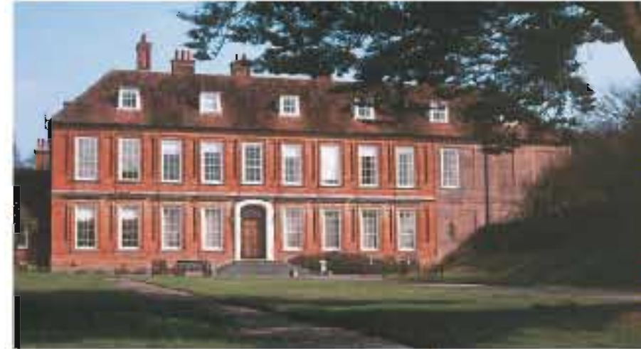
Fine C17th brickwork (Bradenham)
