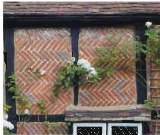
Timber framing with herringbone brick infill (Monks Risborough)
