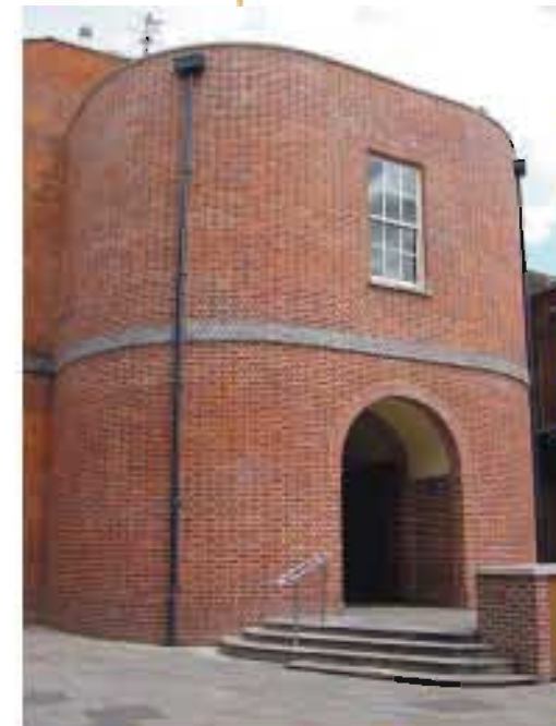
High quality specifications, well executed brickwork together with design flair and imagination are essential to produce brickwork of a sufficient standard to blend in with the region's rich heritage (High Wycombe)
