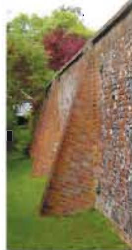
Brick buttresses (Stonor)
