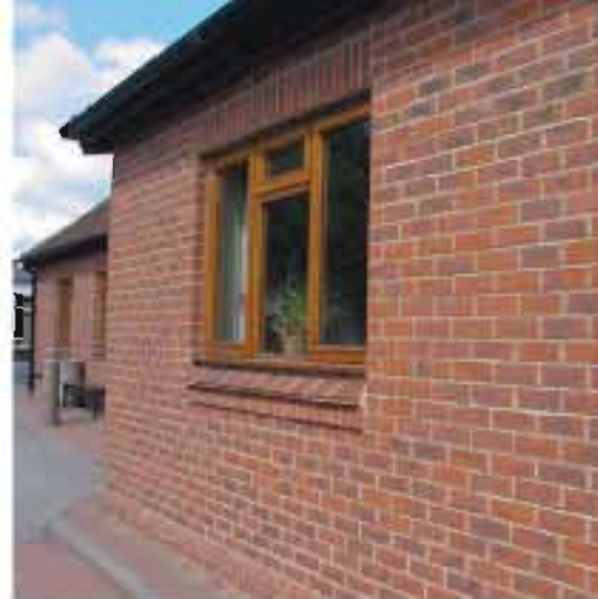
Modern brickwork is usually constructed in stretcher half bond
