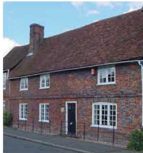
Brick was the favoured material for many smaller domestic buildings of the C17th and C18th (Monks Risborough)
