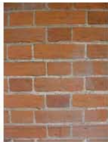
Example of chalky, gritty mortar laid in even beds and finished flush. Note the stack marks on some of the bricks (Ewelme)
