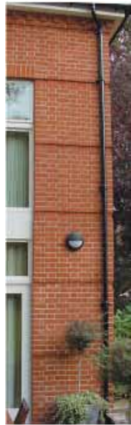
Recessing used to create panels
