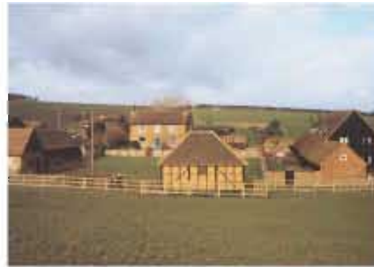
Variations in the bricks and brickwork contribute to the richness of the region's buildings (Chalfont St Giles)
