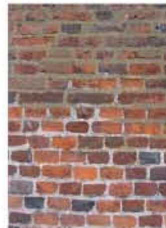
Avoid using hard cement mortars for repairwork
