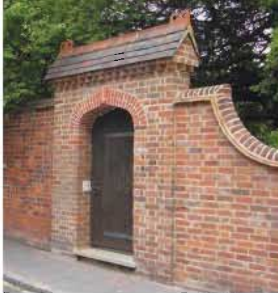
Elaborately swept and capped wall (Marlow)
