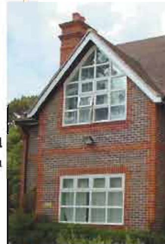
Three course quoin brickwork (Marlow)
