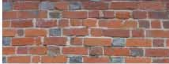
Gritty chalk-rich mortar used in wide joints (Britwell Salome)
