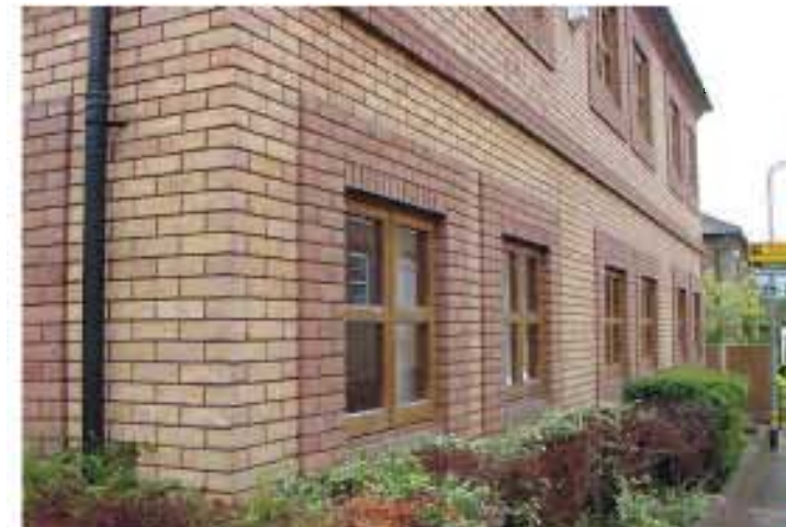
Bland modern brickwork
