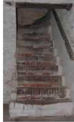
Brick cellar stair (Bledlow)
