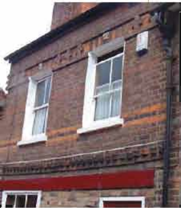
Quirky projecting platband. Note also the treatment of the brickwork above the windows (Great Misenden)
