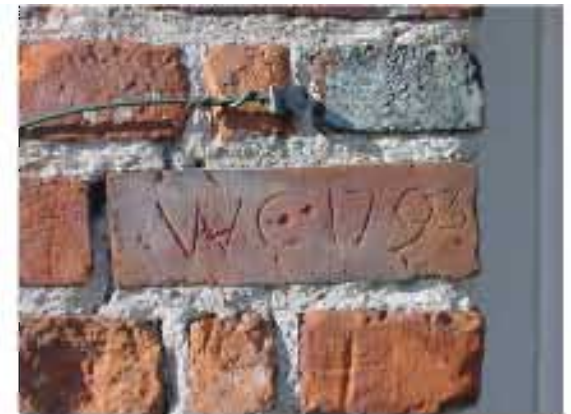
Dated brick (Bledlow)
