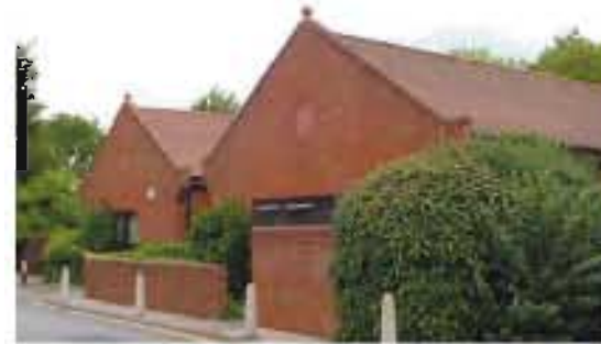
Despite detail being included brickwork can create a monolithic appearance, as here (Tring)
