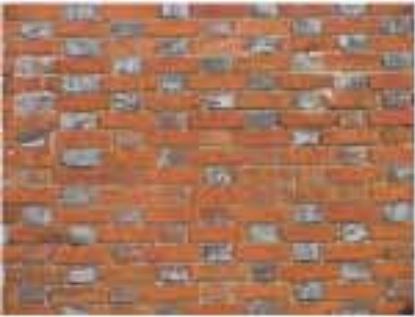
Chequered pattern using burnt headers in Flemish bond (Nettlebed)
