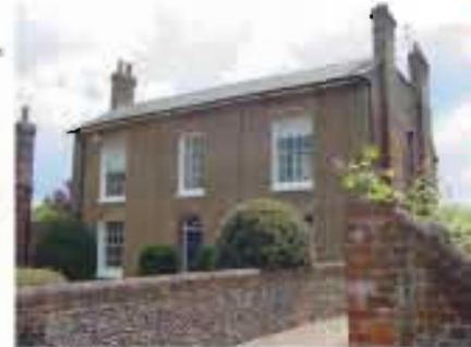
Yellow 'stocks' imported into the region, more prevalent in the north-east Chilterns
