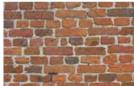
Random bond in C15th brickwork (Ewelme)
