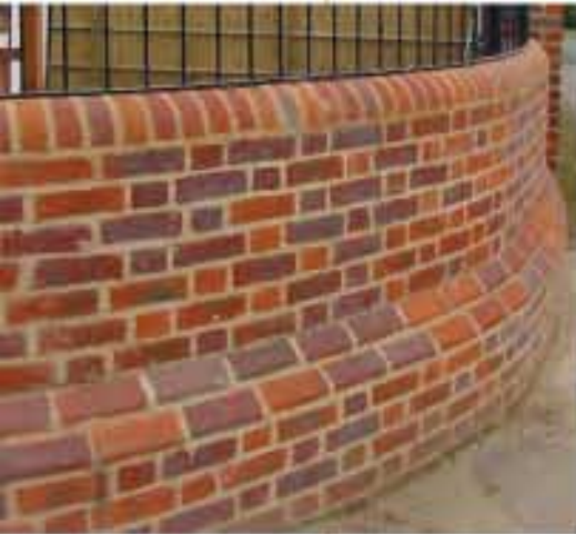
Specials used in plinth (Hemel Hempstead)
