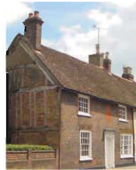
Timber-framed building refronted in brick (Markyate)
