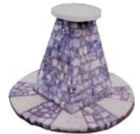
Sundial base of knapped and squared flint (Stoke Row)
