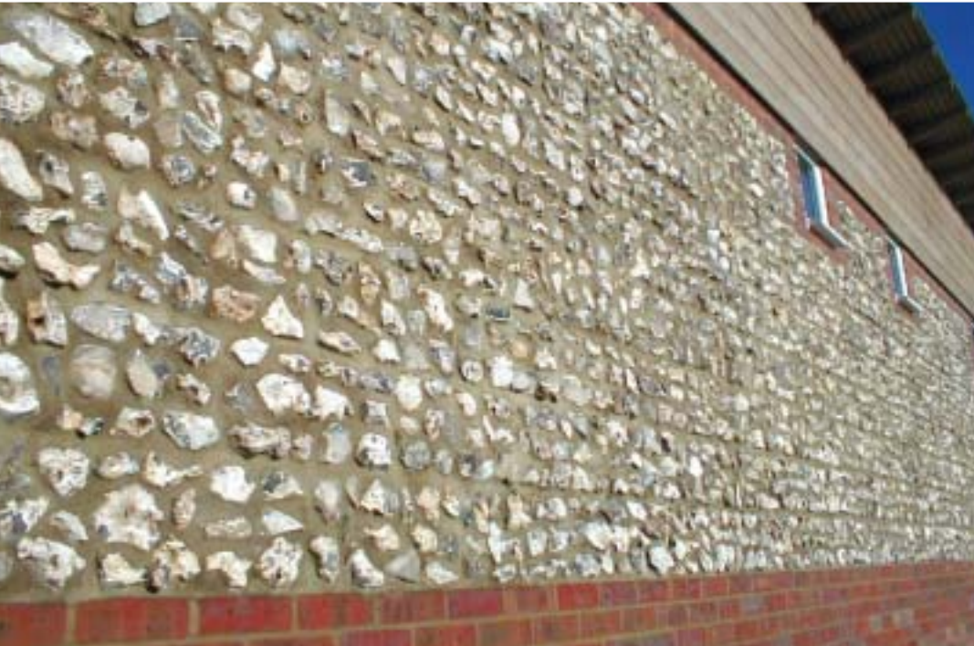
Even with careful pointing the appearance of the banding effect of manufactured blocks is difficult to disguise
