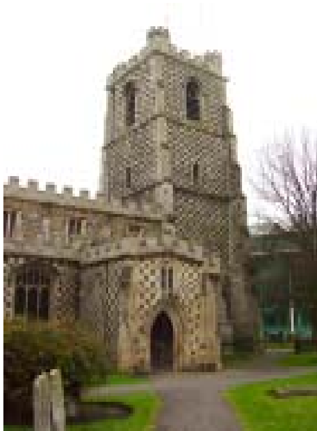
Chequerwork with knapped flint (Luton)
