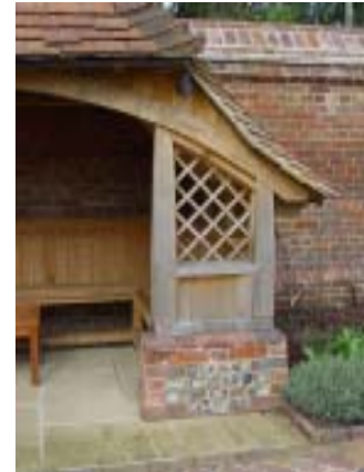
Garden shelter (Chipperfield)
