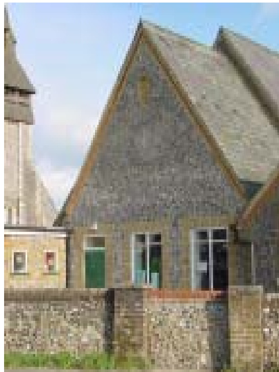
Extension to Chorleywood School
