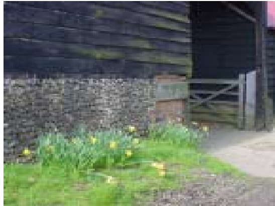
Farm buildings (Kensworth Corner)
