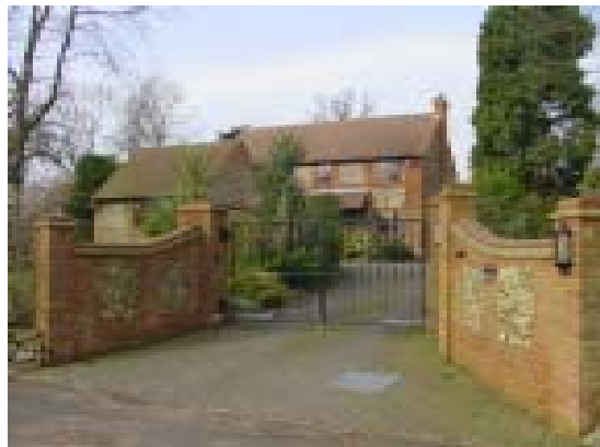
Suburban details look out of place in a rural setting
