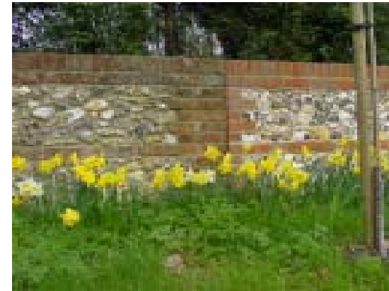
Brick-on-edge capping
