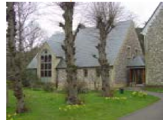
New Church Hall (Chipperfield)
