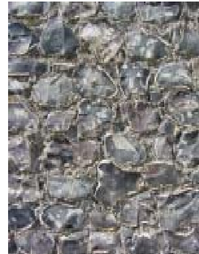
Knapped flint with gritty lime mortar
