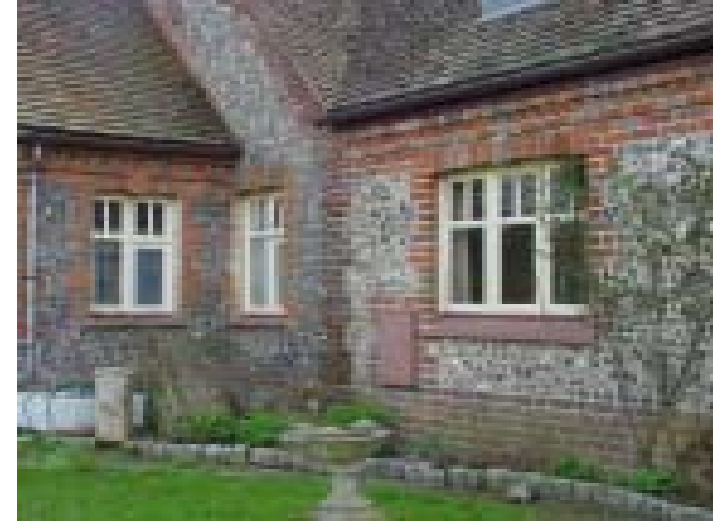
Extensions should be carefully blended into existing flintwork
