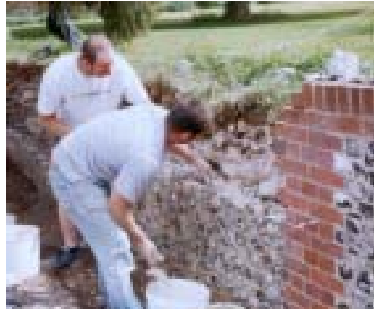
Wall under construction using lime mortar
