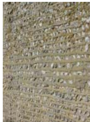
Ribbon pointing swamping original flintwork
