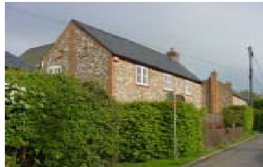
Well designed new flint buildings should dovetail into the surrounding landscape and settlement pattern (Great Kingshill)
