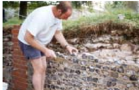
Constructing flint freehand
