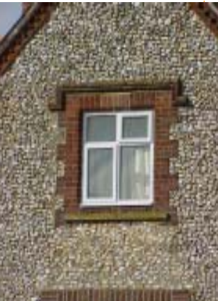
Window with label mould and three-course brick quoining
