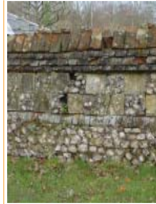
Highly elaborate boundary wall
