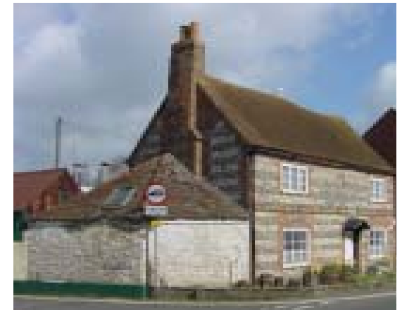
Banded flintwork is only found on the south-western fringes of the Chilterns (Benson)
