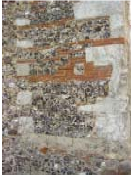
Tiles used in flint and stone buttress
