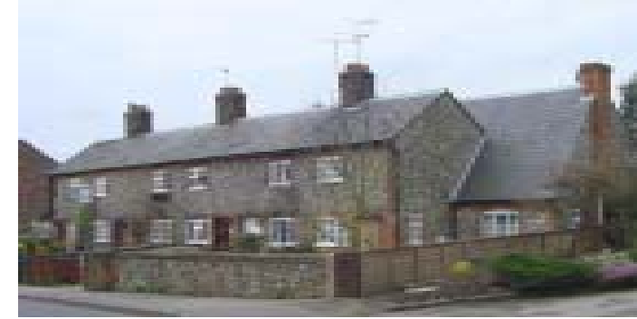
Terraced housing (Woodside)
