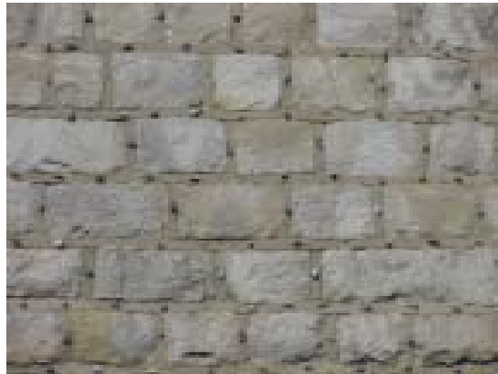
Galleting is seldom encountered in Chilterns. This rare example at Wycombe Abbey shows flint gallets pressed into the mortar of a masonry wall
