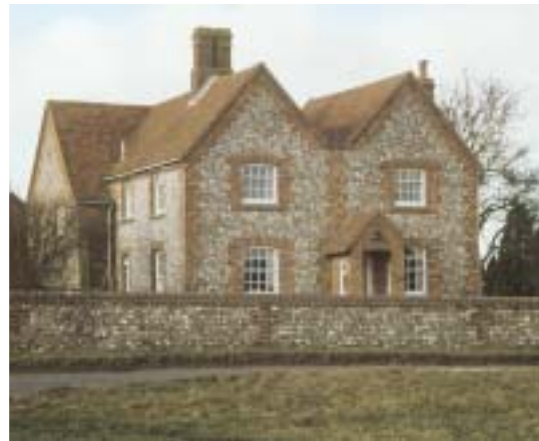
The nineteenth century was the heyday for flint and brick (Wheeler End Common)
