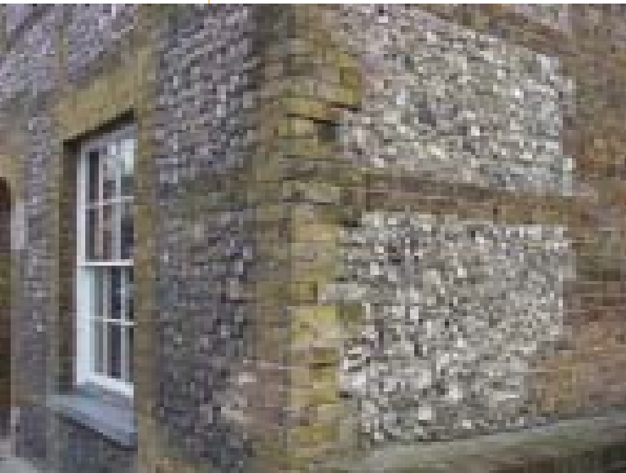
Flints graded by type, size and finish
