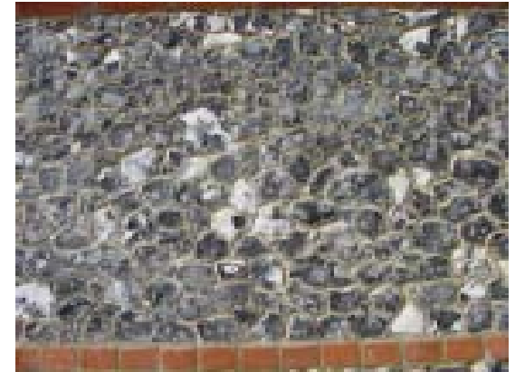
Good mortar finish
