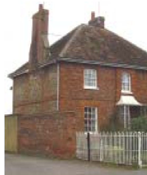
Early C19th brick front, flint side walls (Chinnor)
