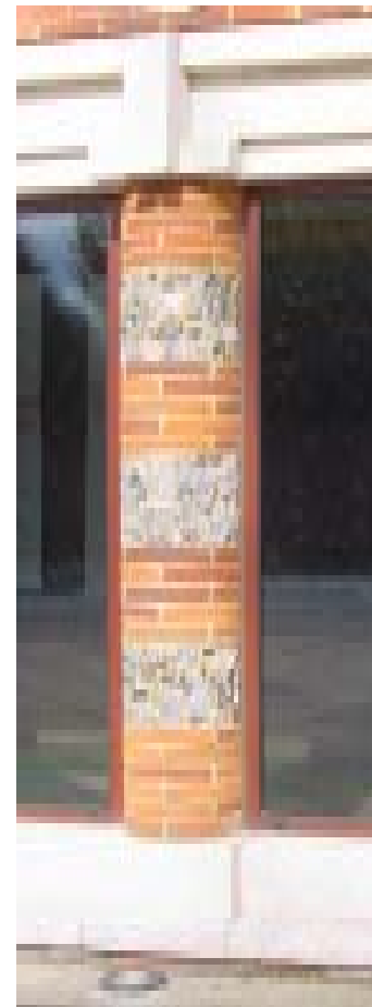
Brick and flint column
