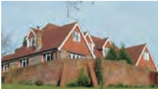
The roof is over-dominant in this low-walled building
