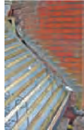
Lead flashings (Hemel Hempstead)
