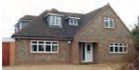
Example of poorly designed steep pitched roof with rooms squeezed into roofspace (Flamstead)
