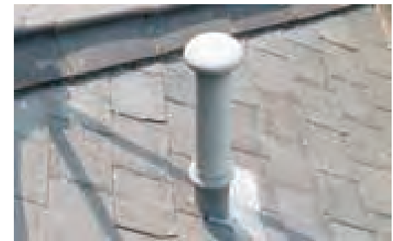
Pipe flashing (Hemel Hempstead)
