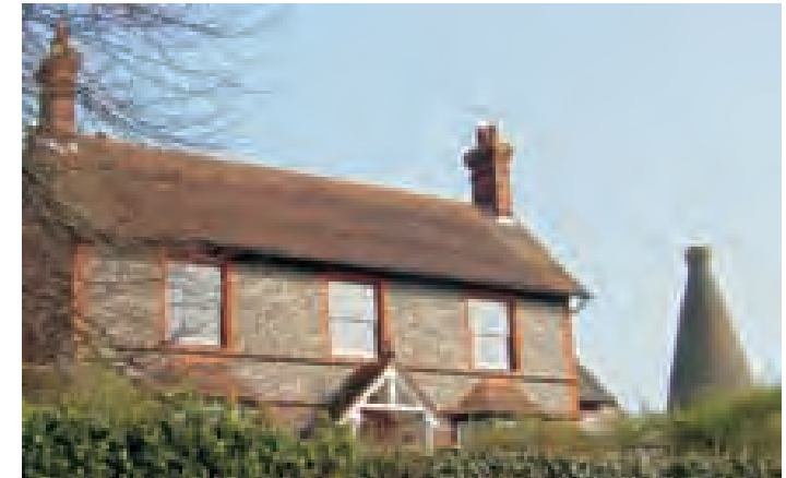
Tilemaking and brickmaking – a decorative tiled roof adjacent to bottle kiln (Nettlebed)
