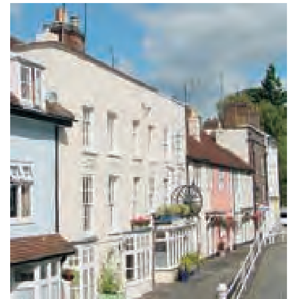
Parapet walls (Hemel Hempstead)
