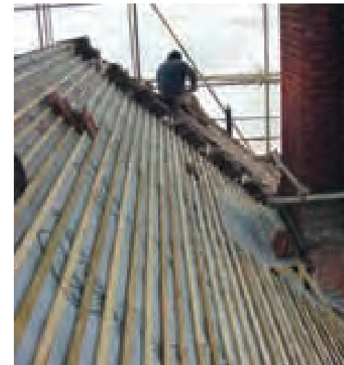
Felted roof (Bury)
