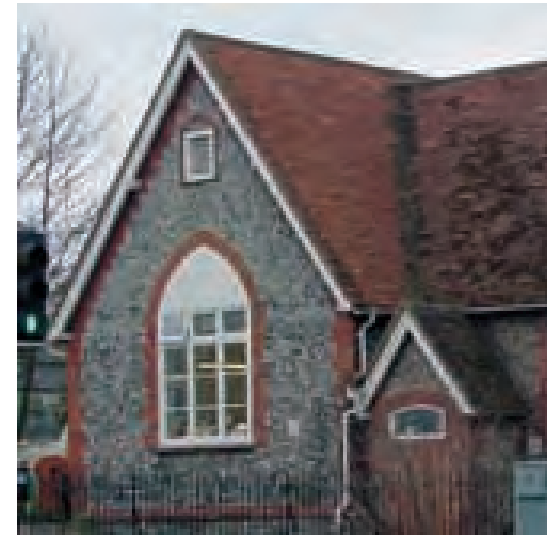
Plain timber bargeboards, echoed on the former porch (Monks Risborough)
