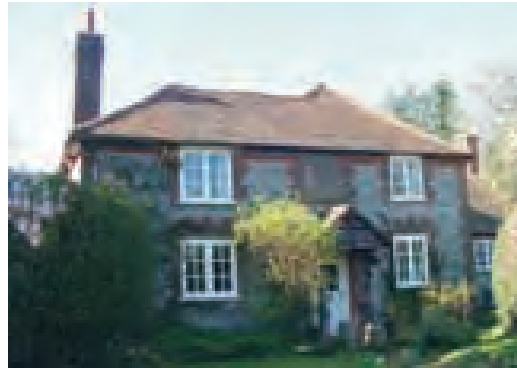
Tiles laid at a very low pitch (Cadmore End)
