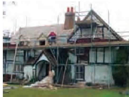
Roof battened out (Brook End Farm)
