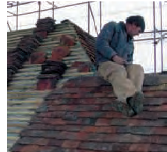
Tiling in progress (Hemel Hempstead)
