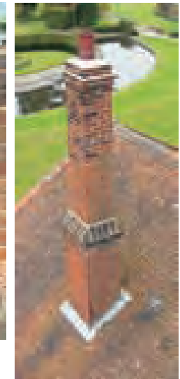
Tall brick chimney, recently repointed (Little Missenden)
