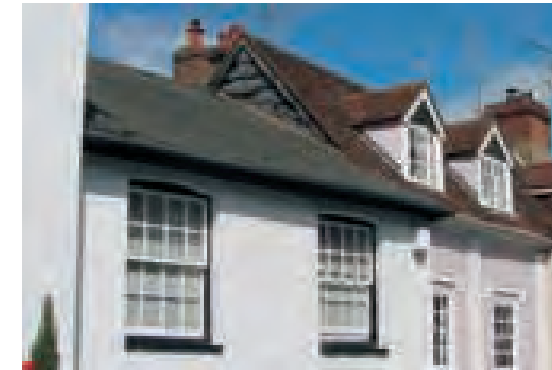
Contrasting pitches for slate and tile (Hemel Hempstead)
