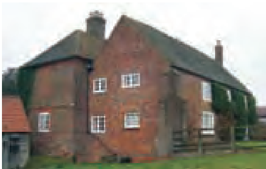
Combined gable and hip (Bledlow)
