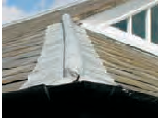
Slate roof with lead rolls (Chiltern Open Air Museum)
