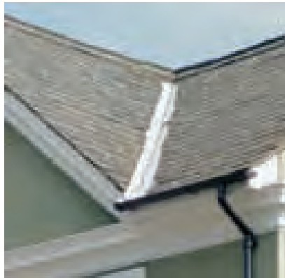
Valley formed in slate roof with metal liner (Berkhamsted)
