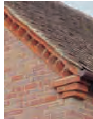
Verge with cogged brickwork (Marlow)
