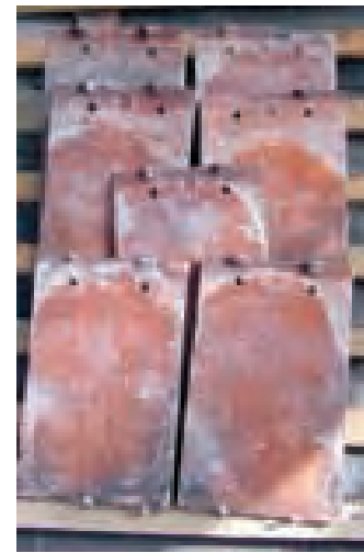
Nibbed tiles (173 High St., Berkhamsted)
