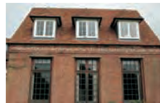
Flat to pitched roof conversion (Christmas Common) (Highly Commended in 2005 Design Awards photos by A. Ingram and C. White)
