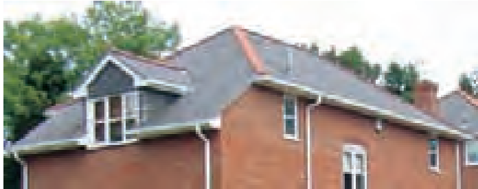
Boxed eaves (Potten End)
