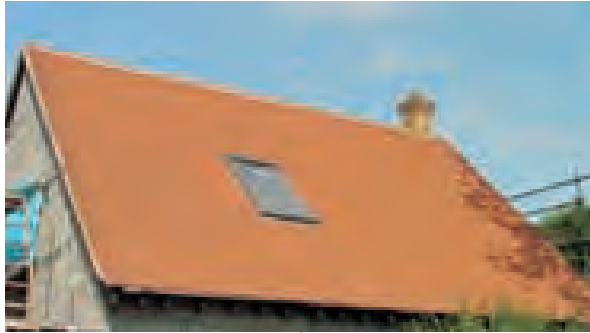
Rooflight in roof of machine-made tiles (Berkhamsted)
