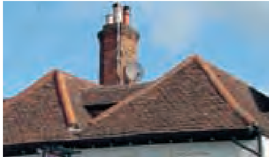
Hip using half-round tiles (Berkhamsted). Note also the intrusive satellite dish and aerial
