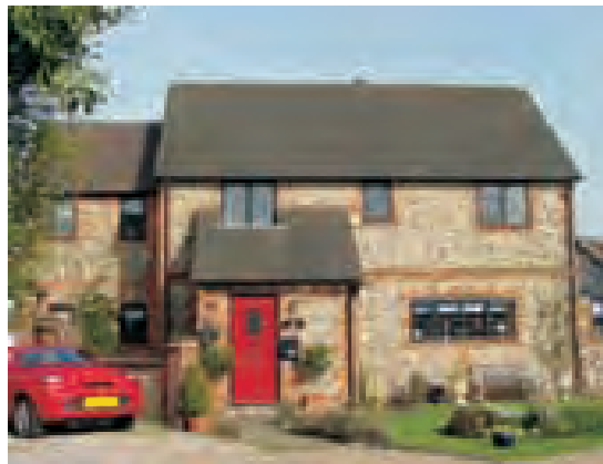
Chimneyless roof (Kingshill)
