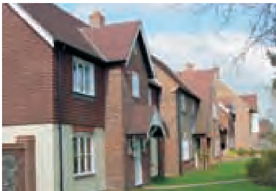
The roof configurations and tile-cladding to this development do not draw on local precedents
