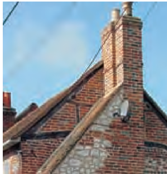
Chimney offset tiled with plain bedded verge to blend in with main roof
