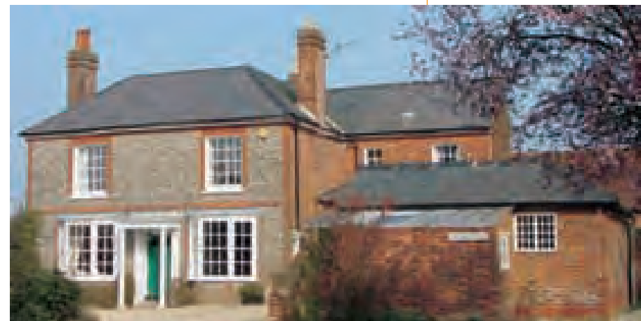
Well executed slate roof (Nettlebed)
