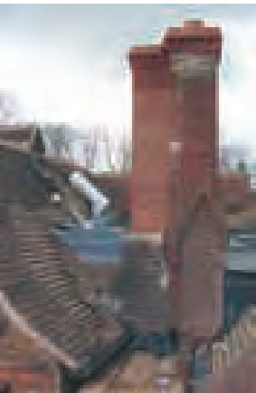
Leadwork to flashings and valley (Beaconsfield)
