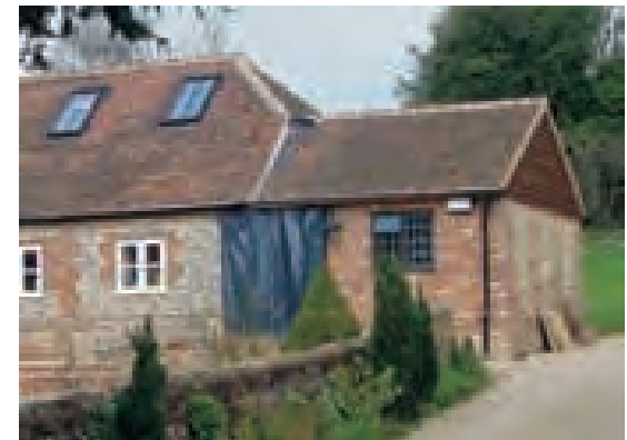
The extension does not tie in with the existing roof shape
