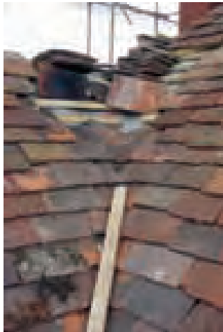
Valley being formed for valley tiles (Hemel Hempstead)
