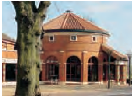
Roof constructed with tegulae appropriate to this Roman site and Museum (Verulamium)
