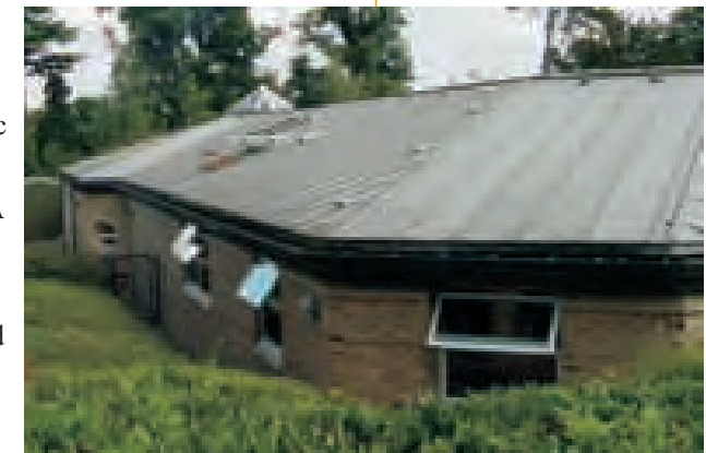
Metal seamed roof (Hemel Hempstead)
