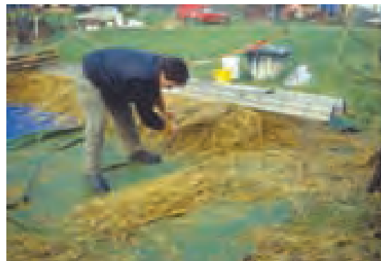
Drawing straw for long straw thatching (Chiltern Open Air Museum)
