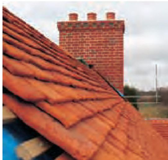
New construction using prototype Chiltern tiles
