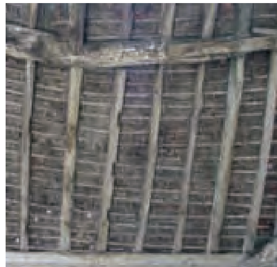
Tiles bedded in straw. Note also the wooden pegs (Fingest)
