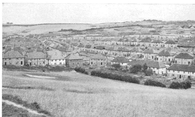
114, 115 BOWERDEAN FARM AND ITS VALLEY, NEAR BEACONSFIELD As they were originally, and as they are after "Development"
