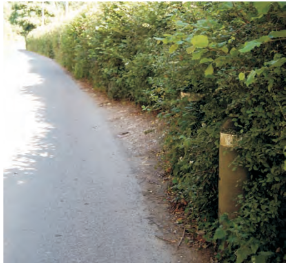
Careful siting of bollards to prevent over running and aid hedge recovery
