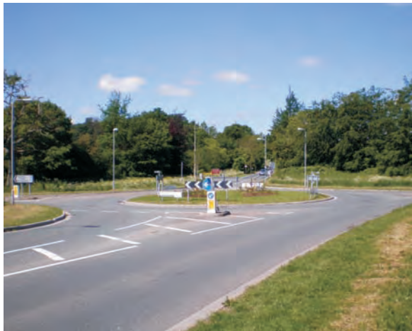
A roundabout where signing and lighting have been minimised - Studham cross roads
