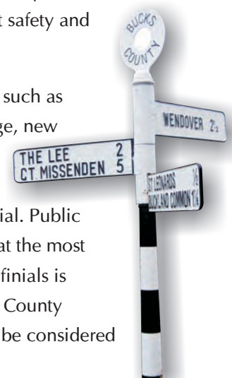
A traditional finger post sign restored with new arm and finial
