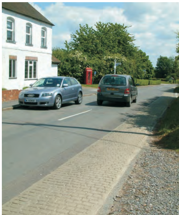
Alternative provision for pedestrians through a village
