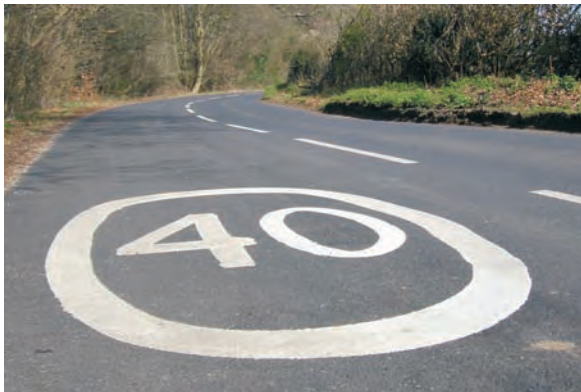
Carriageway signing is preferred to upright signing (which requires Department for Transport authorisation)
