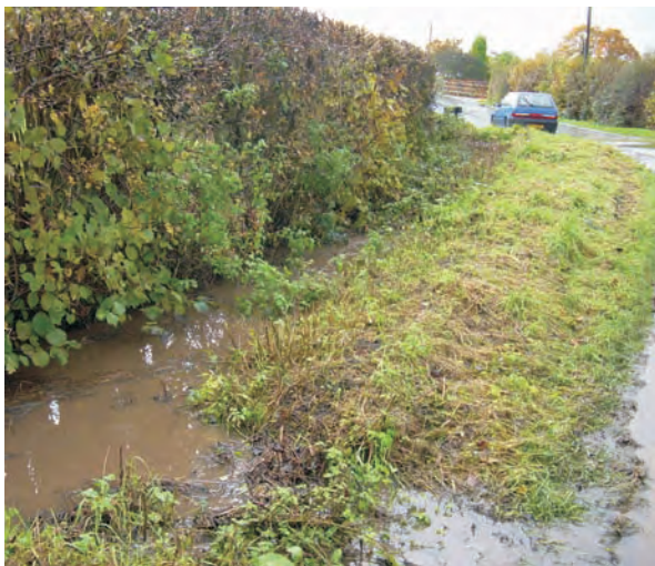
Roadside drainage needs to be maintained
