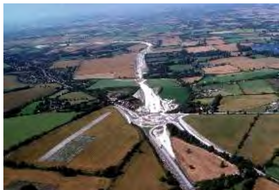
A41 road improvement and bypass, Aston Clinton
