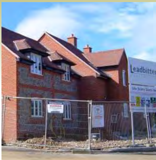
Affordable Housing under construction at Winchmore Hill, Bucks
