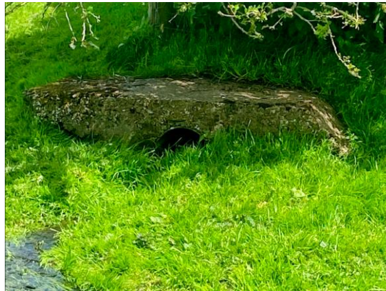
Figure 7 - Image showing the outfall pipe that may connect with the roadside gullies on Valley Road
