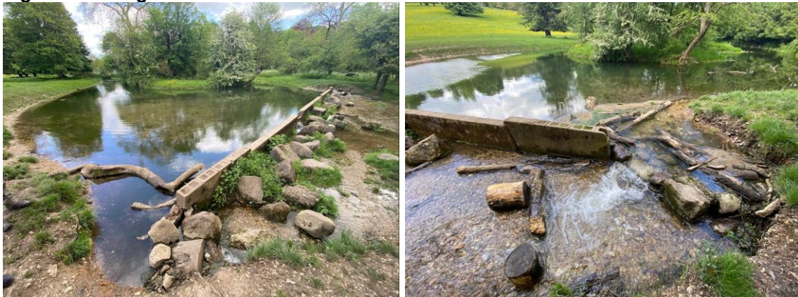
Figure 23 - Images of Weir F. Note that water outflanks the weir at both ends
