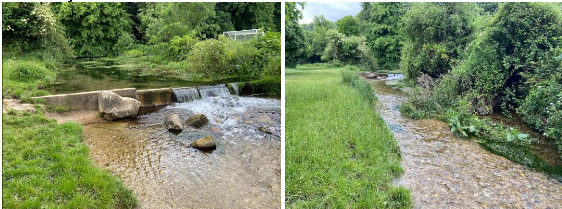
Figure 13 – Images of Weir B that creates the large lake and the elongated riffle that sits immediately below.
