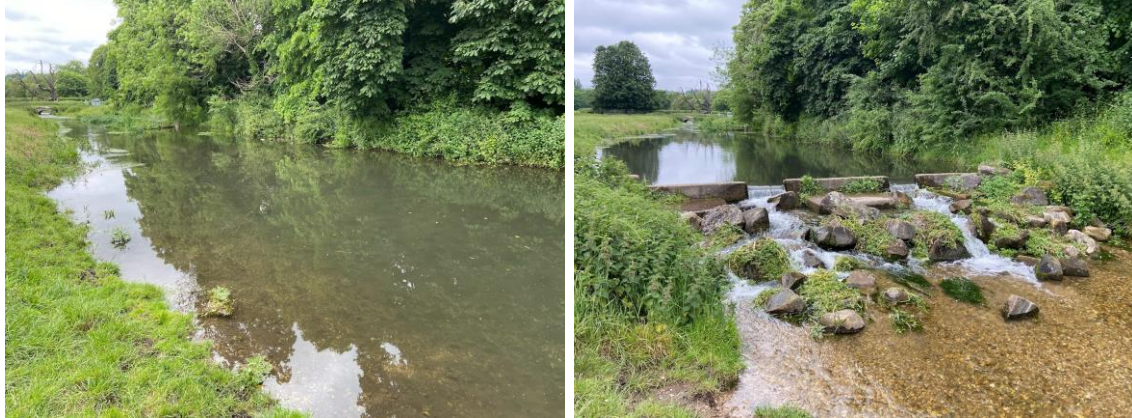
Figure 11 - The first weir on the estate together with the pool it was designed to create
