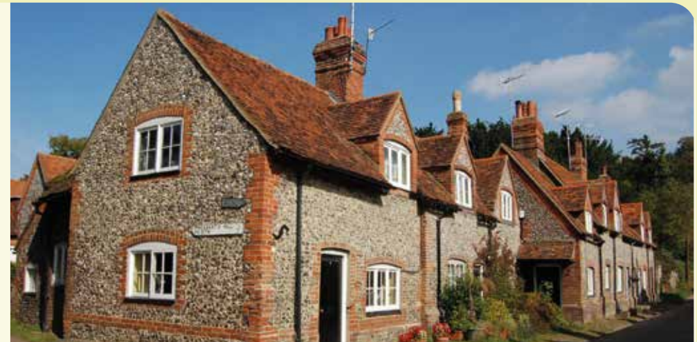
Classic Chilterns vernacular architecture at Turville: small-scale cottages of local brick and flint with clay tile roofs.
