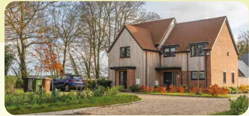
New development at South Stoke, Oxfordshire
