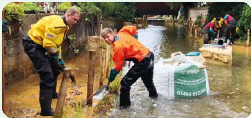
Volunteers restoring a chalk stream
